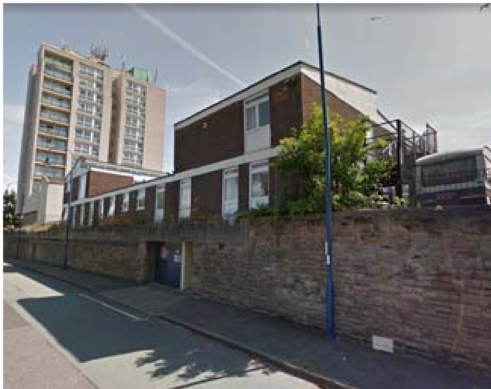
Rear Elevation – Note basement car park entrance.
