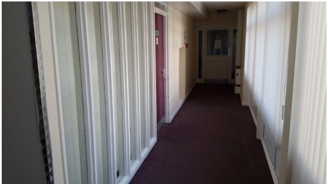
Photo. 5 – General view along GF corridor.
