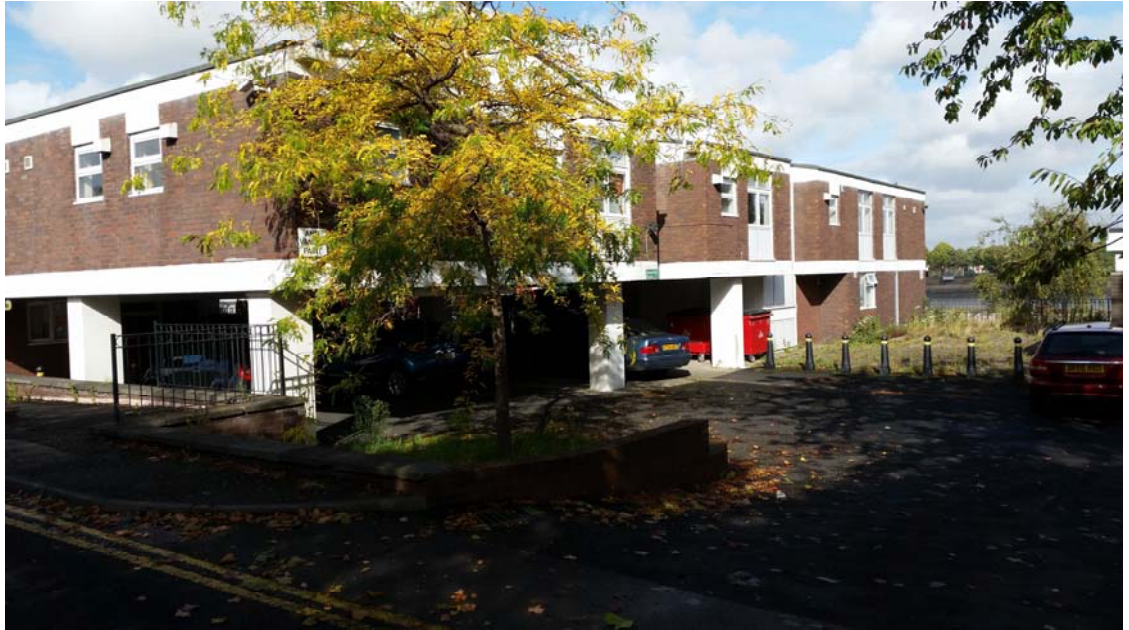
Photo. 1 – General view of Belvedere and car park.
